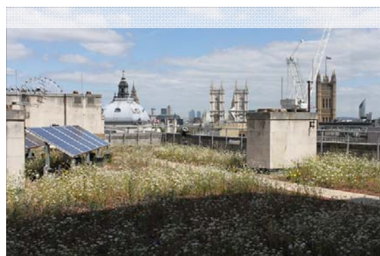
Above: Transport for London HQ (Green Roof Consultancy)
