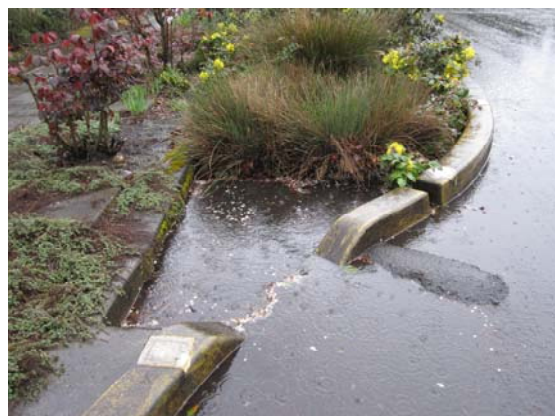
Below: Rain garden, Portland, Oregon (Dusty Gedge)
